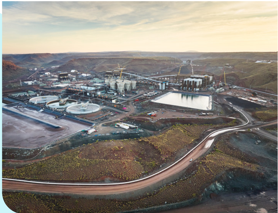
Iron Bridge Project
